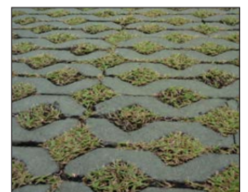
Below: Low-impact materials include turf block that allows water to get through to sub soil instead of washing off ground surface.
