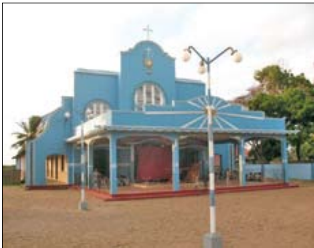
Figure 3.7 – St. Mary's church, Arippu (Sampath Goonatilake © IUCN)
